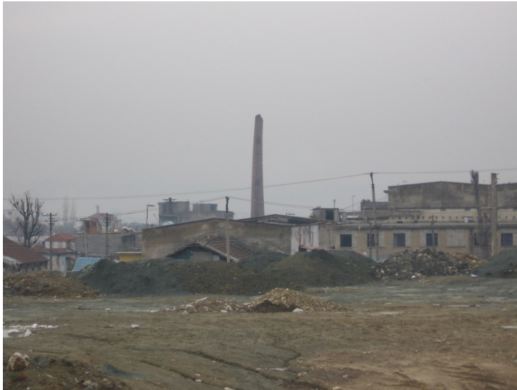
Figure 29: Figure of the old tractor factory (preparation of construction)
